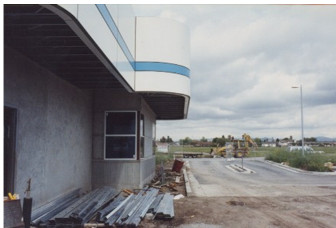
This is the MOA facility while under construction. When it was finished in 1991, LAVTA was able to relocate from outdated facilities in downtown Livermore. However, the agency has again outgrown its property and is in need of a satellite facility to complement the existing premises.
